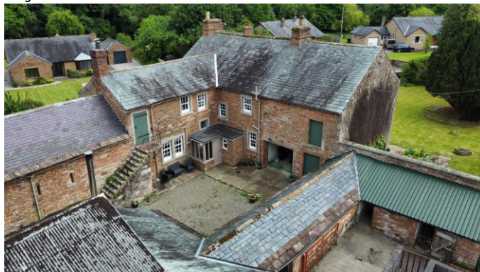
Wythmoor House – Rear Elevation
