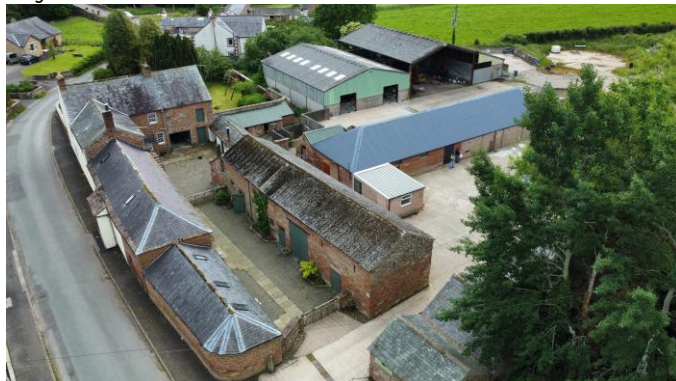
Wythmoor House – Rear Elevation
